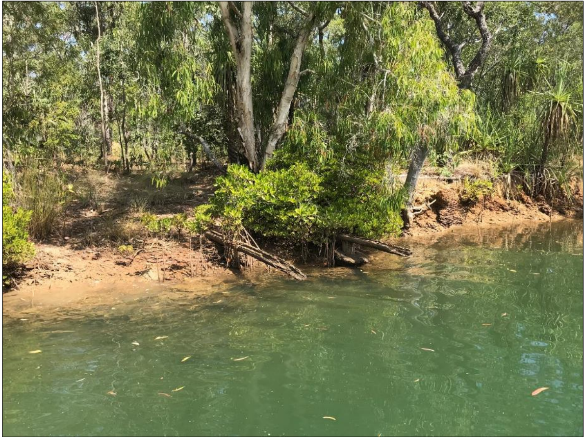
Figure 6: Remnants of the jetty and boat slip on the Emerald River - part of the original Mission built in 1921 (coordinates: 136.441711°, -14.079216°)
