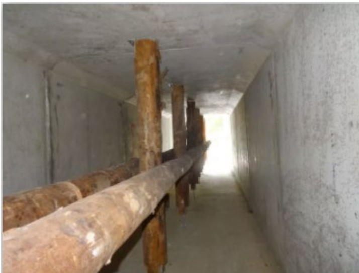
Figure 2: Example culvert style underpass for critical weight range ground dwelling fauna.
